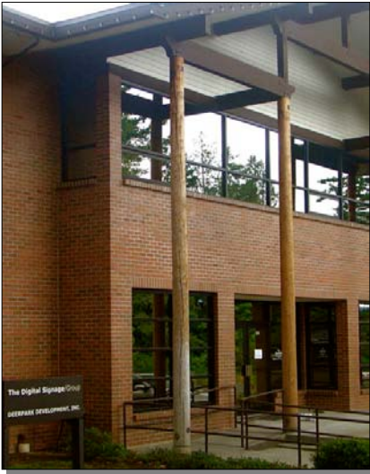
Building at Powder Hill Business Park
